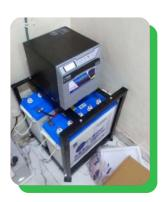
A key component for the energy transition is energy storage given the intermittent nature of renewable energy sources. The energy stored in the batteries serve as back up when the grid power is unavailable. In the course of 2024, Solfa Power installed energy storage systems of about 75kwh capacity of energy storage as back up to customers who had existing solar systems
