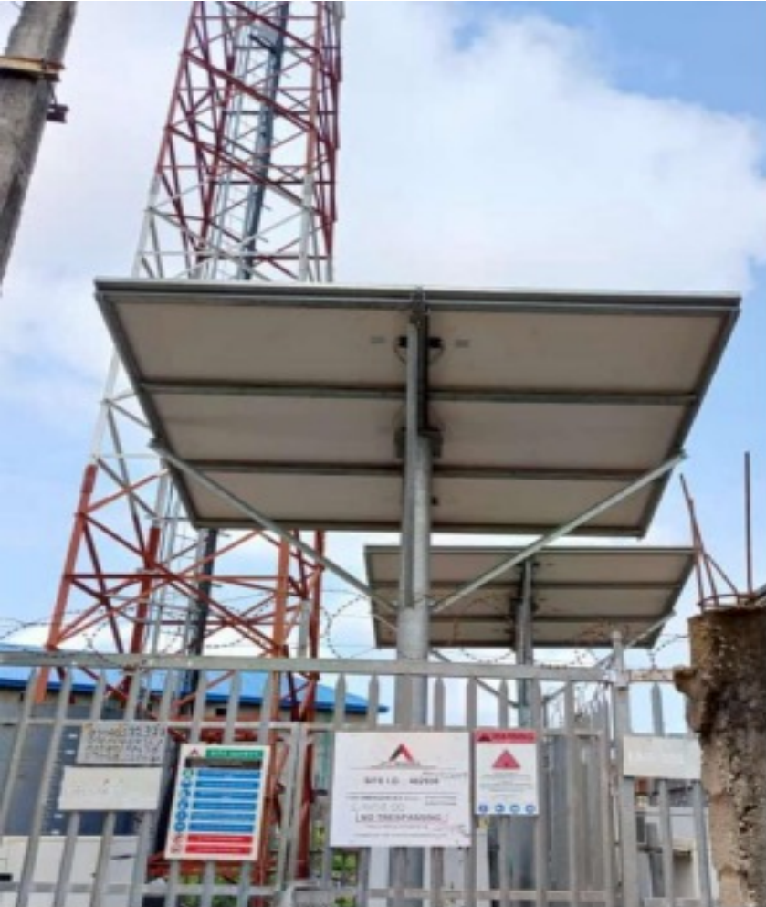
SOLAR INSTALLATION FOR A NETWORK MAST
